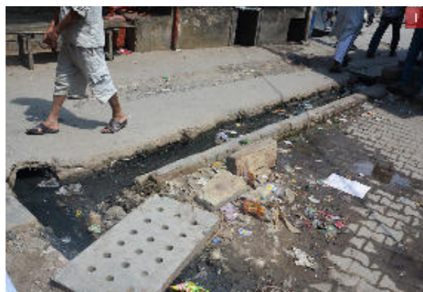
Open Sewer Line at Madipur Village
