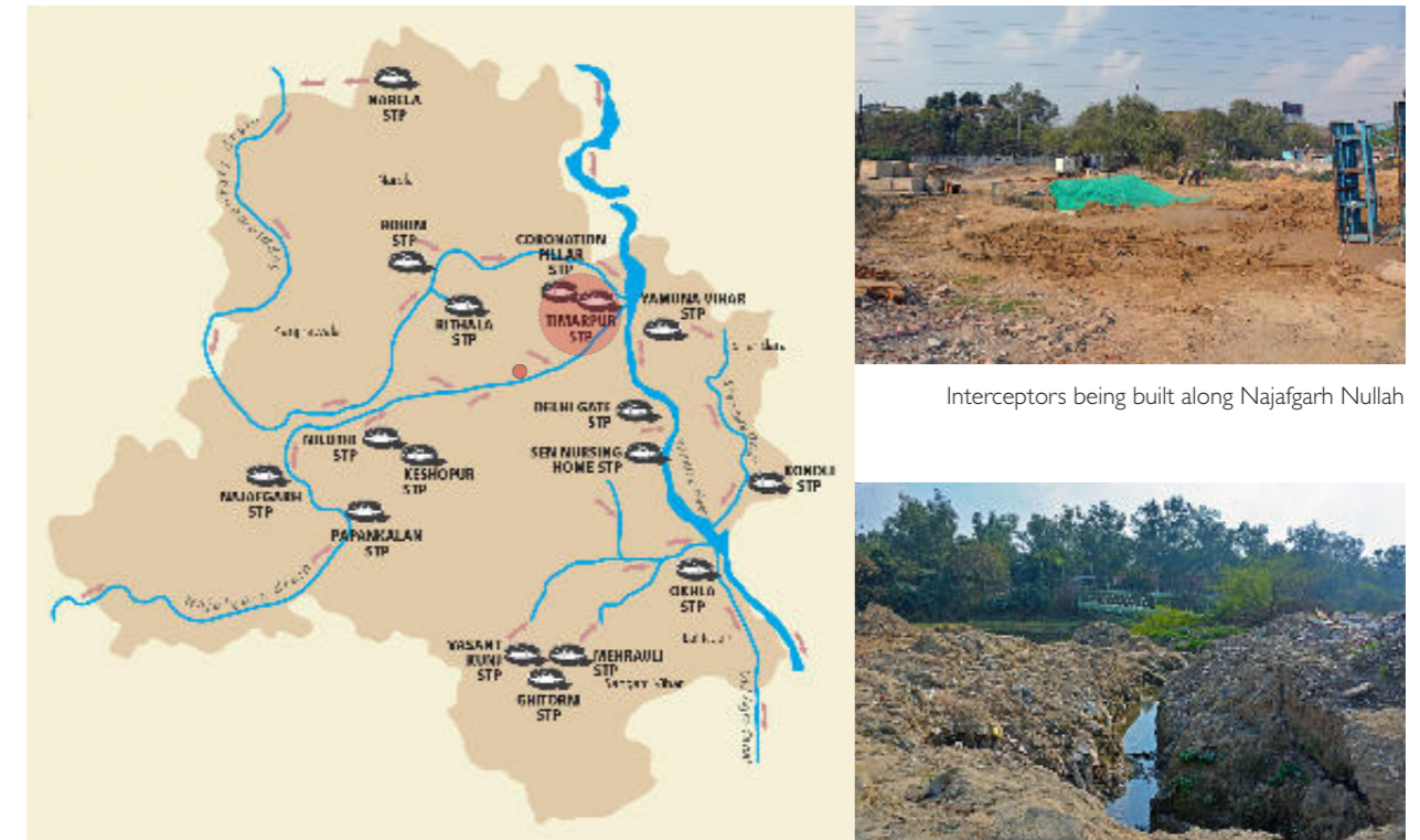
Sewage Treatment Plant with respect to Ward 103
