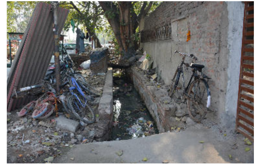
Condition of drains
