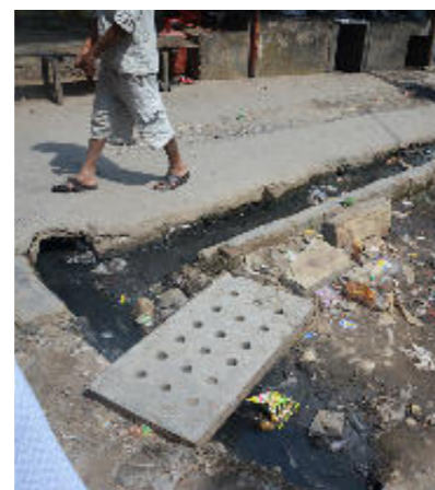
Condition of stormwater drain
