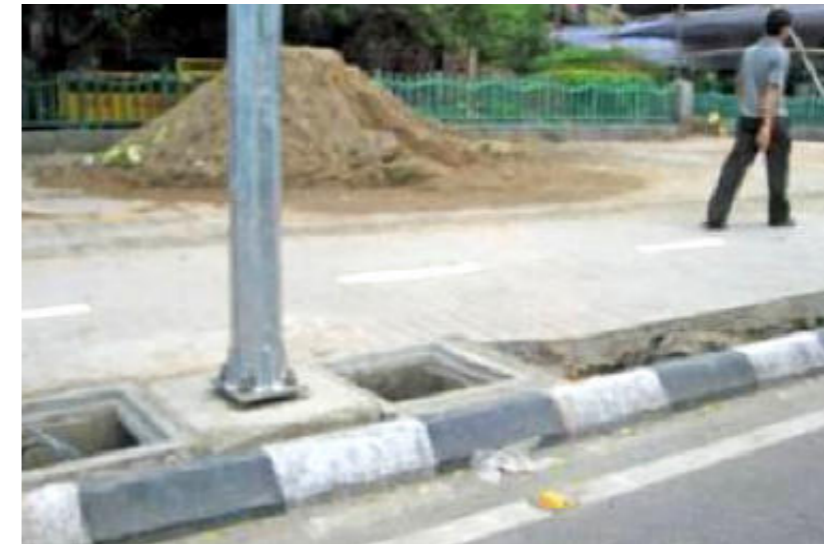
View of fully accessible CUD (Source: UTIPEC Streetscaping guidelines, 2009)
