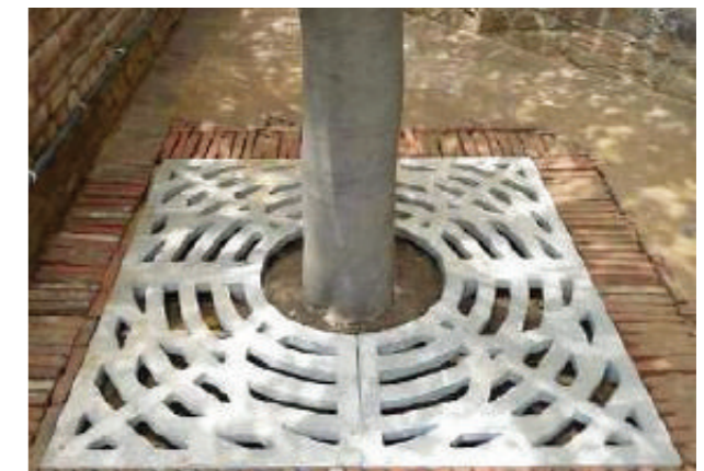
Precast cement concrete tree grate (Source: UTIPEC Streetscaping guidelines, 2009)
