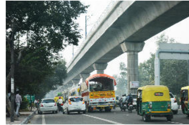
No proper lane division
